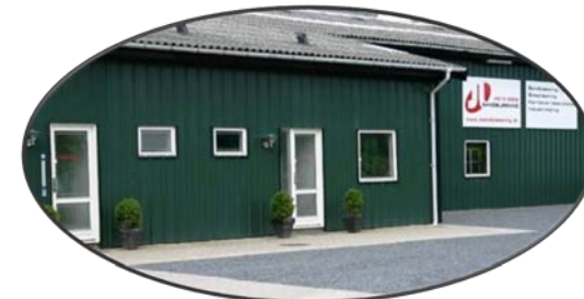
Free energy checks for industries
