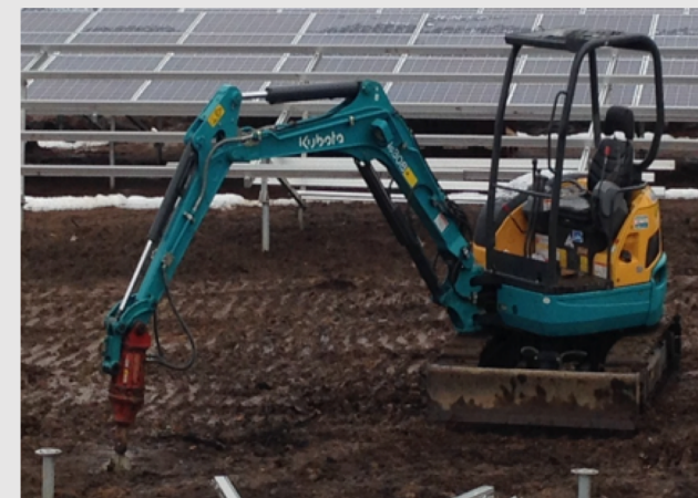
Sample of a drilling machine in Japan
